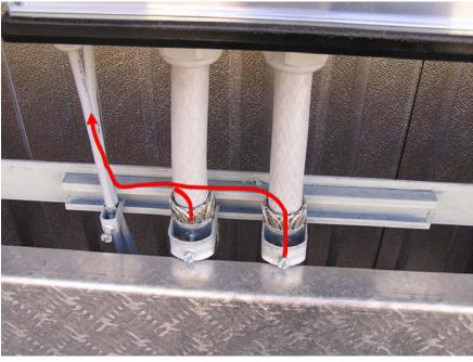
Bus communication interrupted due to noise coupling to communication cables
