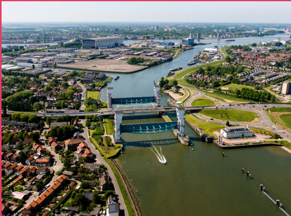
Figure 1: The Hollandsche IJssel storm surge barrier
