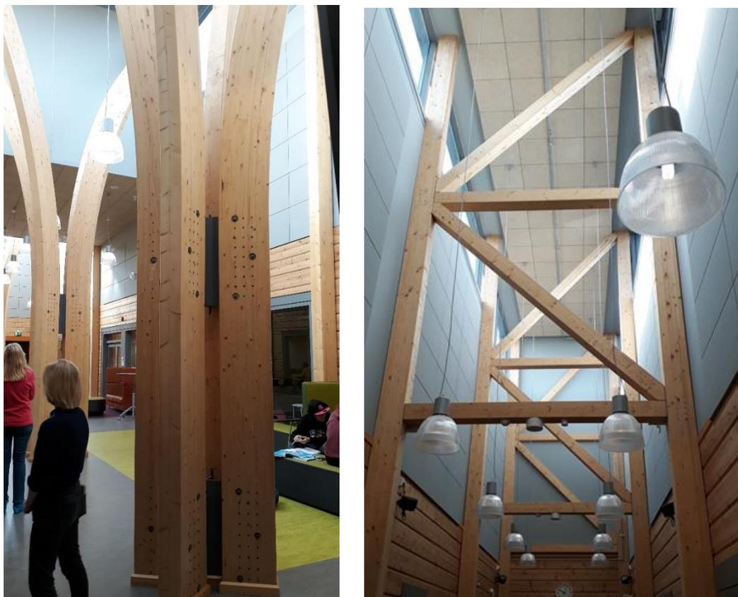
*Pictures 10-12. Roof support structures of a log campus (pictures by Virpi Palomäki, CE Wood -project)*
