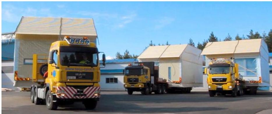
*Fig. 20. The modules are removable with the foundation. Photo by Teijo-Talot Oy*
