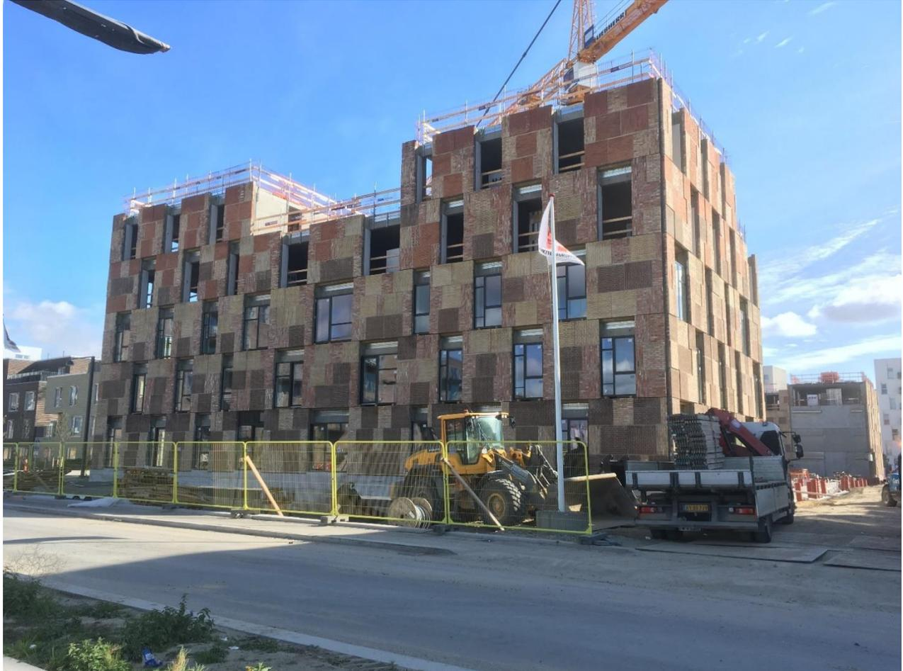
*Pictures 2. The bricks for The Resource Rows are cut out in modules and stacked up to create the new walls of the building. There are also recycled wood based materials from the Copenhagen Metro construction. (Picture by Virpi Palomäki and Paula Pihlaja, CE Wood -project)*
