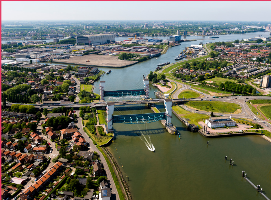
Figure 1: The Hollandsche IJssel storm surge barrier. Courtesy RWS, mediatheek.
