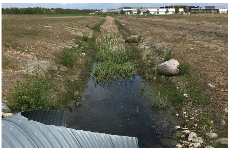
Figure 3 Study-site 2 (looking upstream), a relatively young two-stage channel restored in 2015. Photos: EA International (March 2019).
