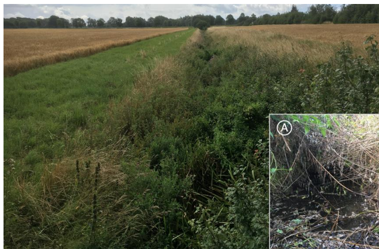
Figure 5 Study-site 4 (looking downstream), a well-established agricultural ditch showing signs of heavy overgrowth. A) close observation shows that vegetation is dominantly from the side embankment. Photos: EA International (August 2019).
