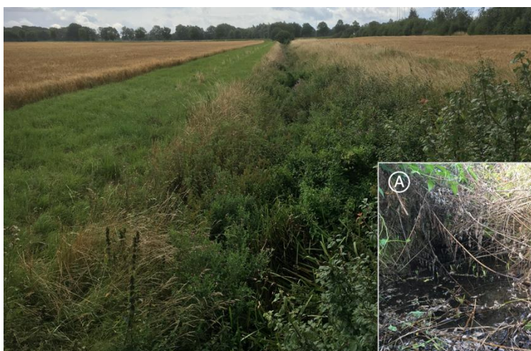
Figure 6 Study-site 4 (looking downstream), a well-established agricultural ditch showing signs of heavy overgrowth. A) close observation shows that vegetation is dominantly from the side embankment. Photos: EA International (August 2019).
