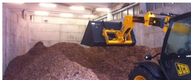
Figure 3. Garliava biomass boiler-house
