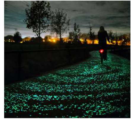
Example 3. An illuminated bike path made out of swirling solar-powered LEDs and light-collecting paint, Eindhoven, Holland https://inhabitat.com/roosegaarde-studios-bike-path-is-a-twinkling-road-inspired-by-van-gogh/
