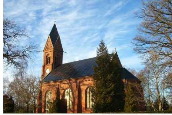
Example 2. photovoltaic on the roof of the church in Greiswald (Dorfkirche- Wieck) https://commons.wikimedia.org/wiki/File:Greifswald_-_Wiecker_Kirche.jpg
