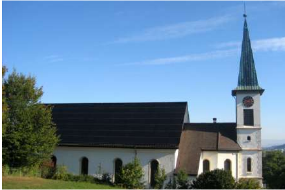
Example 1. Frameless photovoltaic on the roof of the church of Saint. Peter and Paul in Ettingen http://www.rkk-ettingen.ch/ueber-uns/kirche-st-peter-und-paul.html ,
