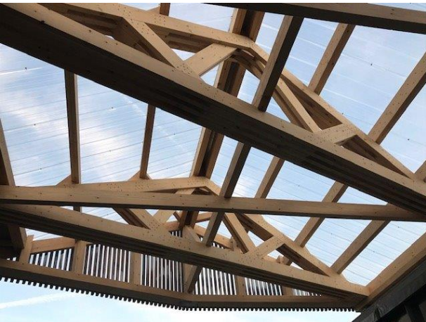
Fig. 15 - Spruce dowelled roof structure at Épinal [U Lorraine].
