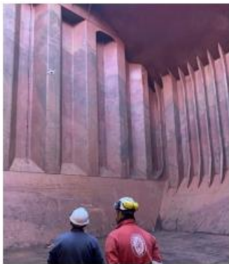
Drone operator with Bureau Veritas surveyor and drone in flight. Image Courtesy of Bureau Veritas.
