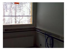
Replaced window in room 260 has improved thermal comfort greatly. There was no air leaks to be found, and overall temperature in and around the window is higher than in 2011.
