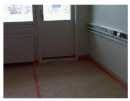
Balcony door has been replaced and now has better air tightness, resulting in better thermal comfort.
