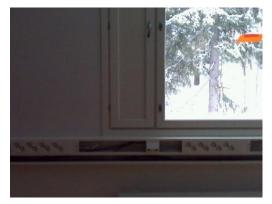
Ventilation window has noticeably better air tightness when compared to the situation in 2011. There were no extremely low temperatures present in 2018.
