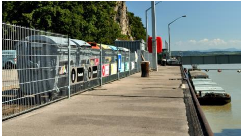
Figure 15: Waste collection facilities at an Austria lock
