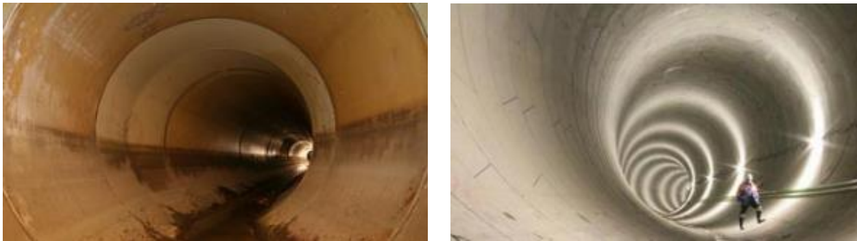
Figure 12: Liesingtal-sewer (left) Wiental-sewer (right) (City of Vienna, 2019)
