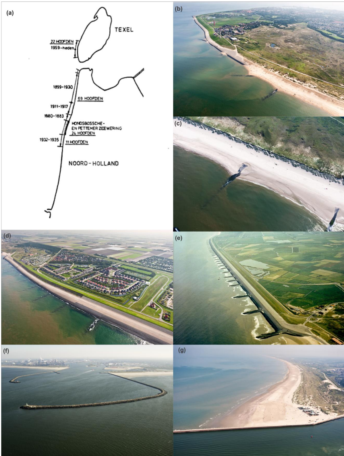
Figure 3: Overview of coastal infrastructure for the Noord-Holland area: (a) construction periods of groins, from: Verhagen en van Rossum (1990), (b) seawall at Den Helder, (c) groins between seawalls of Den Helder and Hondsbosche-Pettemer, (d) Hondsbosche and Pettemer seawall in 1982, (e) south end of Hondsbosche and Pettemer seawall in 2011, and (f,g) harbour jetties of IJmuiden and sedimentation on the north side in 2011. Images from: https://beeldbank.rws.nl , Rijkswaterstaat. Source entire figure: Deltares, 2017
