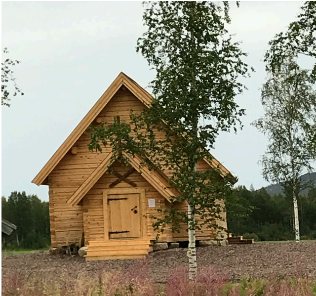
The Särkilahti Chapel, which was destroyed in a extreme spring flood in 1671, north of Ylitornio, has been rebuilt next to the Northern Lights Route.
