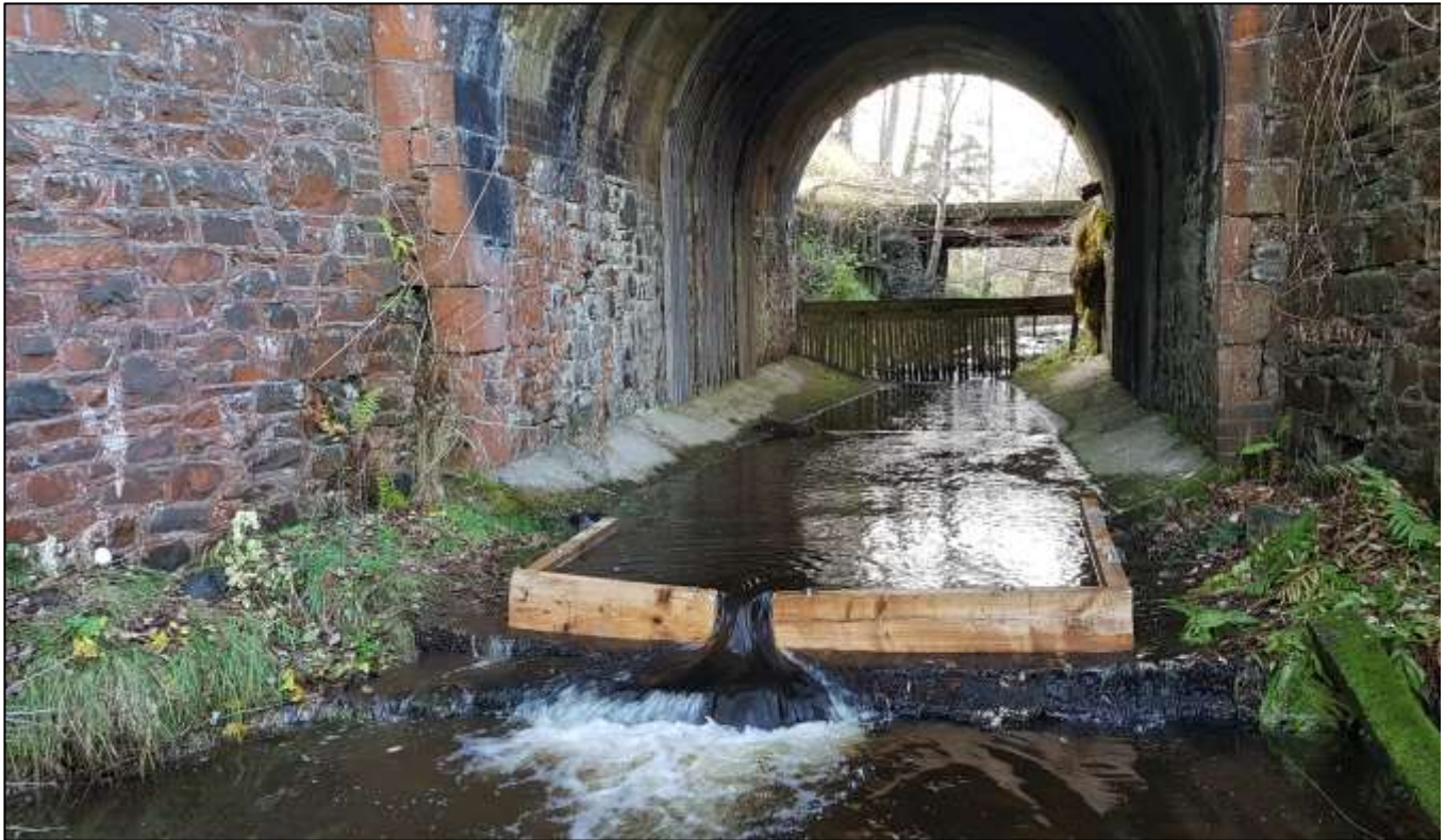
Figure C5b. Weir with wooden fish pass installed pre-autumn 2018
