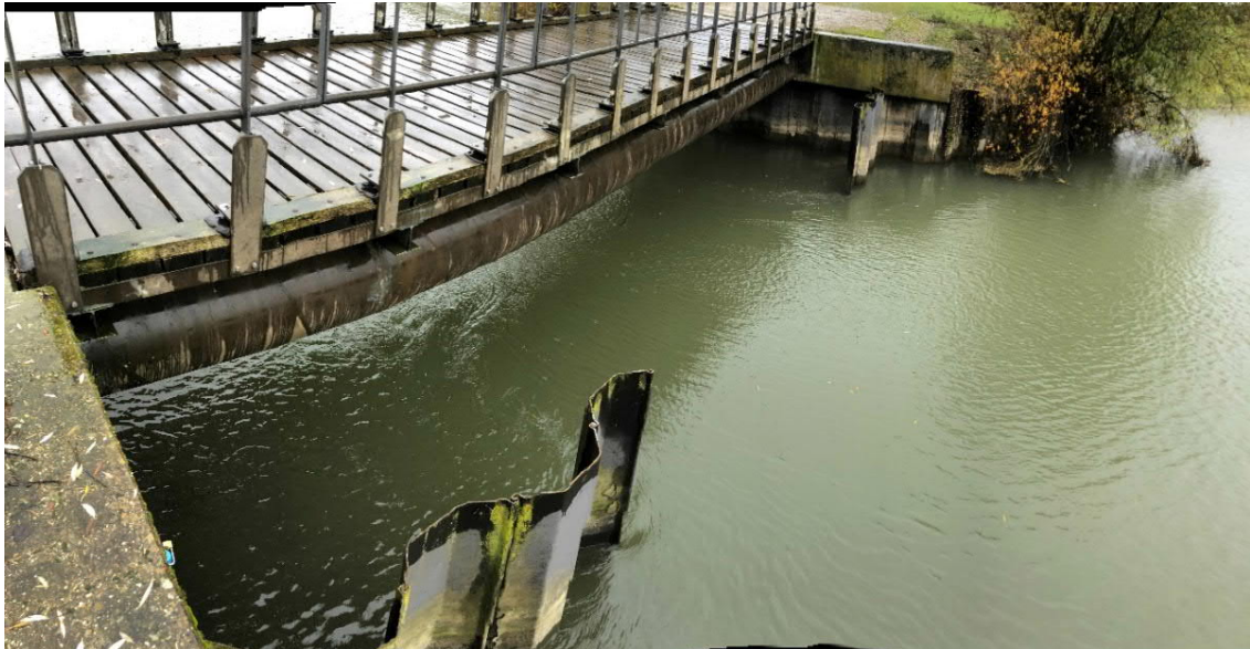
Figure 3.26 Gamerensche Waard: bridge over inlet construction with narrowing of the flow.
