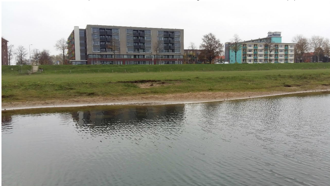
Figure 3.72 Zandweerdhaven: slight erosion on the east bank (November 2019).
