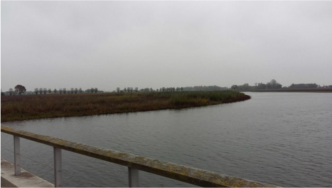
Figure 3.78 Duursche Waarden: southern channel (Olster floodplains), constructed in 2015. This channel only flows at exceptionally high river flows (once every 10 years), no morphological dynamics are to be expected here.
