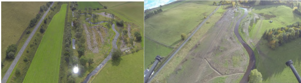
Figure 6 Two of the re-meandering measures, implemented in the Eddleston catchment area.
