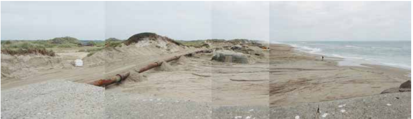
Figure 14 Beach nourishment performed at Krogen/Krylen in September 2008.
