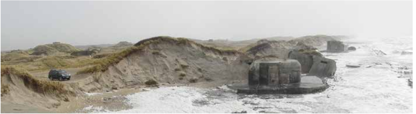
Figure 9 Picture from Krogen/Krylen right after an acute erosion event in March 2008.
