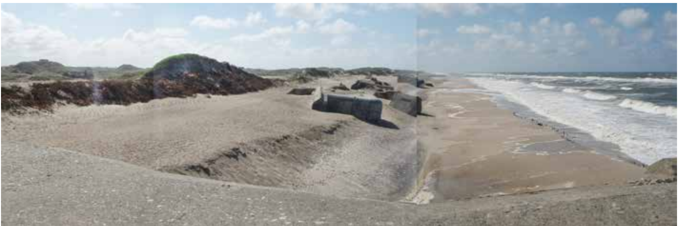
Figure 15 Beach nourishment at Krogen/Krylen photographed in May 2009, a year after nourishment.
