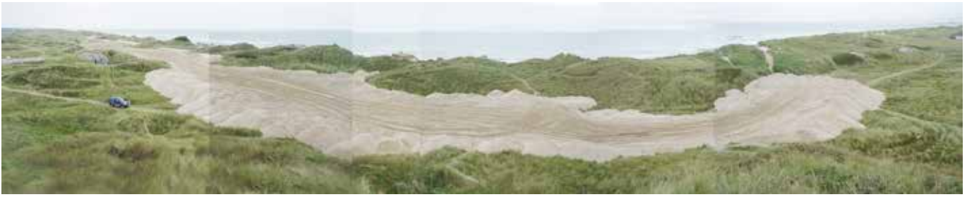
Figure 13 Dune reinforcement performed in September 2008.
