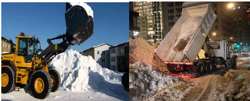
Figure 2.3 Loading and Disposal of Snow
