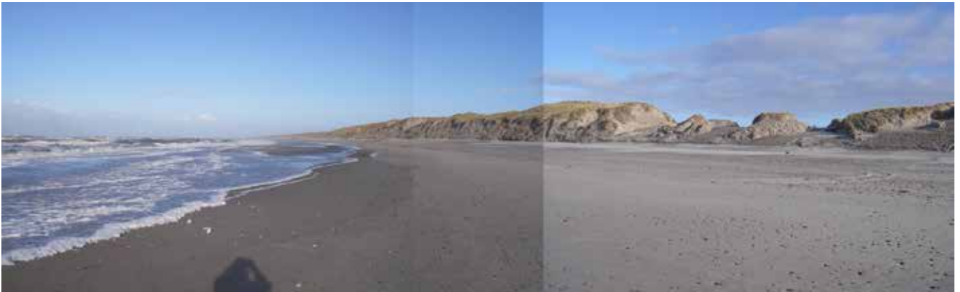
Figure 10 Photo from Skodbjerge on January 7 2007. The dune front is eroded over a long stretch and there is a local breach.
