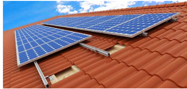
Pic. 2.27: Set up of PV modules on roof with special holders
