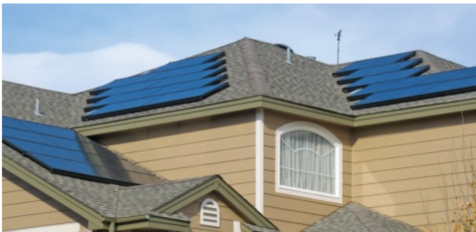
Pic 2.3: PV panels placed on roof with different pane azimuth and plane tilt
