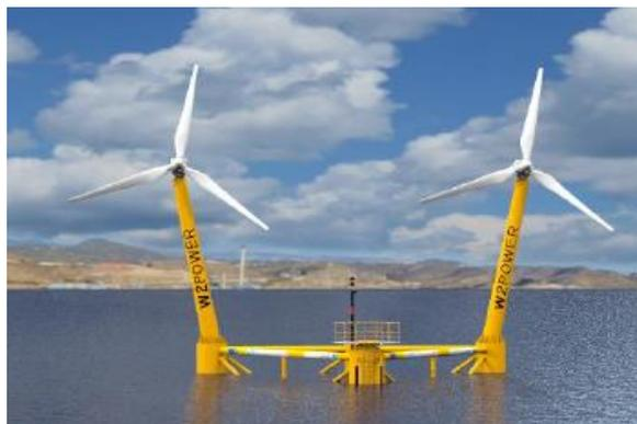
**ENEROCEAN - W2POWER:** Prototype floating Wind power platform
