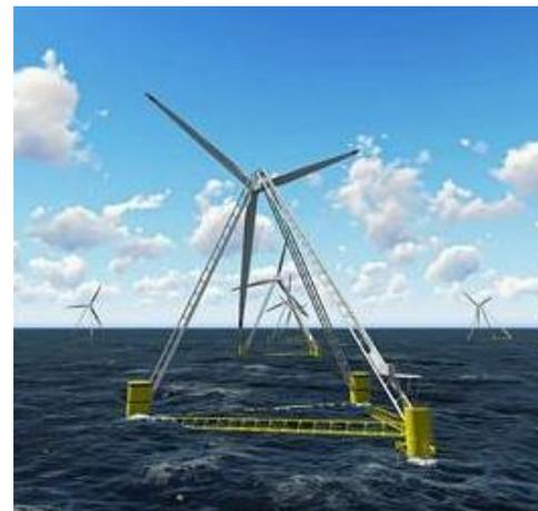
**X1 WIND – PivotBuoy:** Prototype floating Wind power platform
