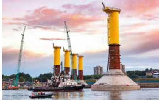
*The first float-and-submerge gravity based foundation being towed on the River Tyne
