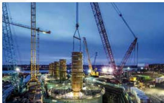
The GBFs have been constructed by Royal BAM Group in the Neptune dry dock on the River Tyne, Wallsend. These concrete and steel structures have been floated into position at sea and submerged onto the seabed to provide the support structures that act as the foundations for the installation of the turbine towers.
