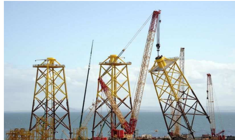
Jacket fabrication at BiFab in Fife
