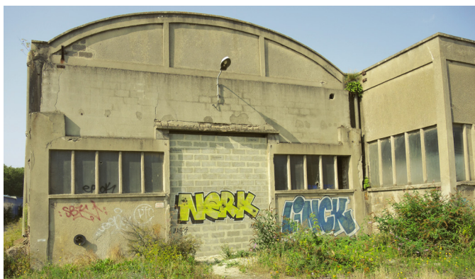
Priority: secure and preserve the building ©MVRDV
