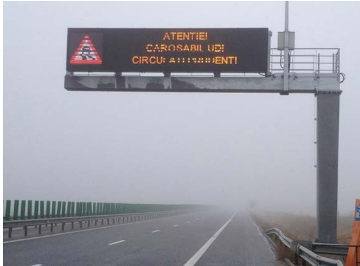
Figure 3-4 Example of a VMS on A2 motorway
