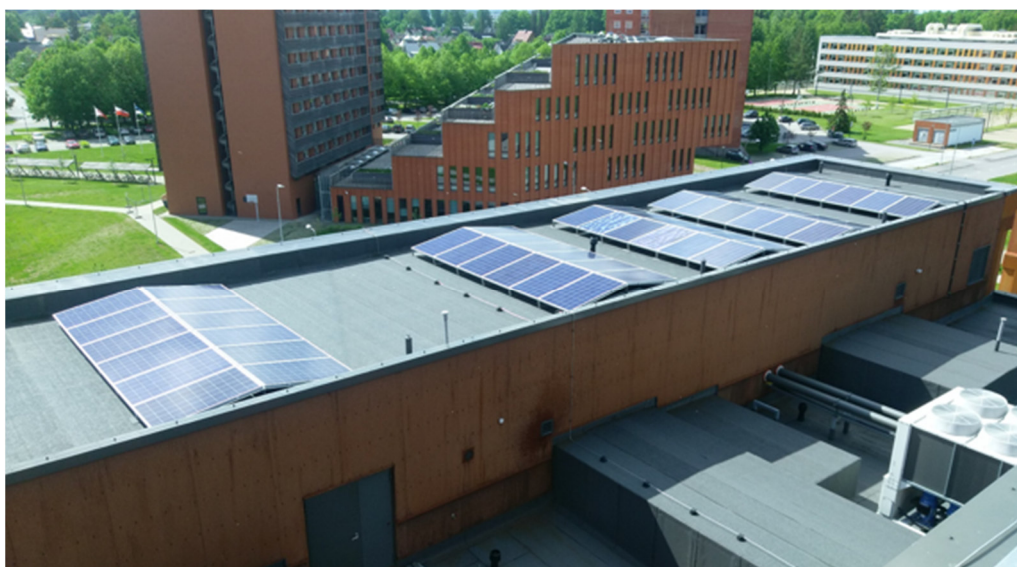
Figure 3: Five PV-test systems on the roof of the Physicum.
