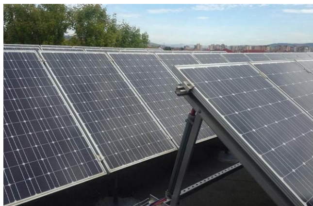
Figure 3: Solar PV Panels installed on an elderly home at Alba Iulia municipality.
