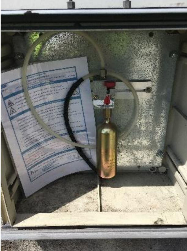
Figure 4: Remotely controlled valve control unit
