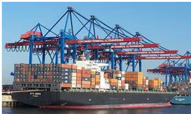
Figure 6 – Hamburg Altenwerder CTA - container terminal
