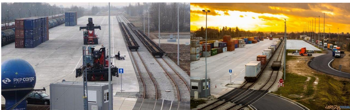
Figure 10 – Poznań Franowo – container terminal
