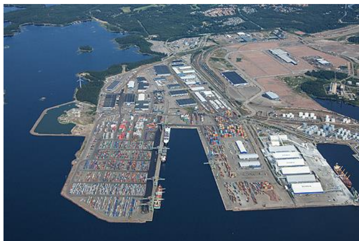
Figure 16 – Mussalo Container Terminal-Kotka
