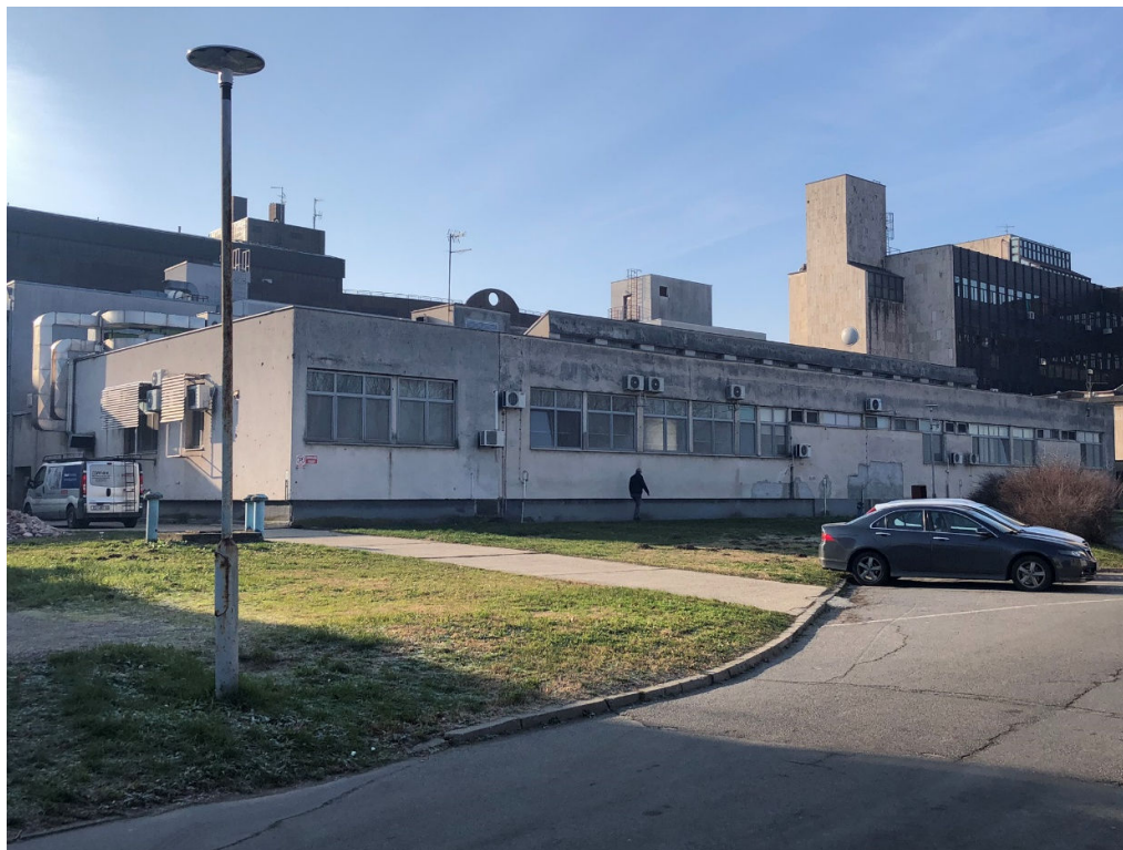
Figure 2.15 North side of the building of Department of Diagnostical Interventional Radiology
