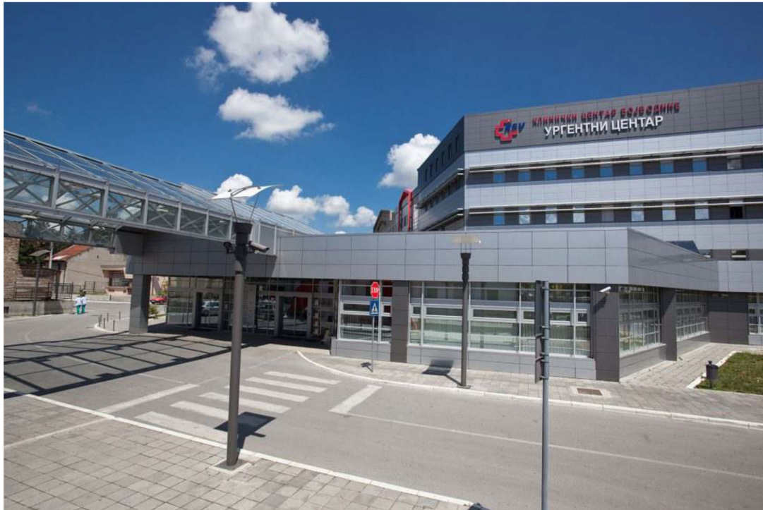
Figure 2.7 Emergency Center facility inside KCV complex
