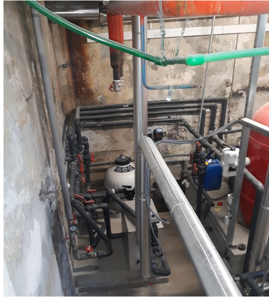
Figure 6.21 Interconnection between solar-thermal and existing heating system
