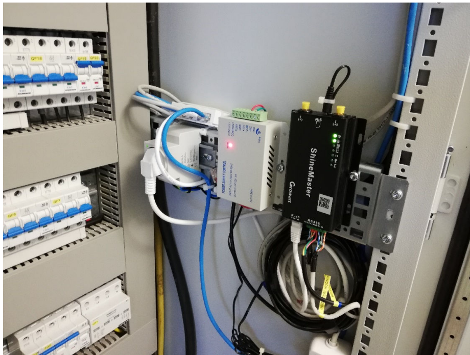
Figure 7.10 FERIT data logger Growatt ShineMaster
