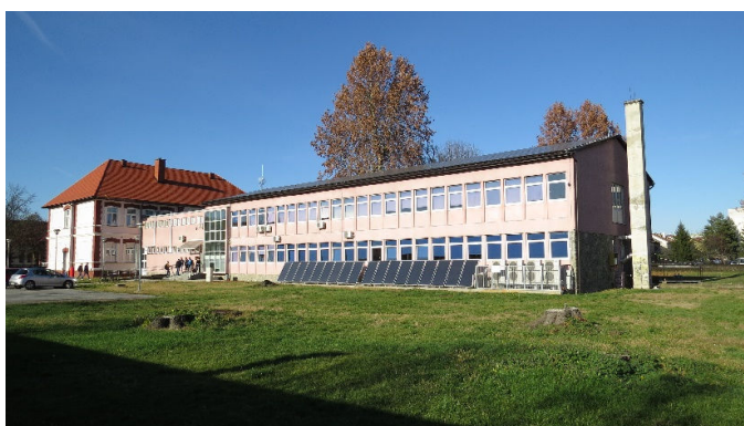
Figure 2.20 Part of Mechanical Engineering Faculty with classrooms and offices where the thermo-technical (solar thermal and heat pumps) system and photovoltaic power plant are installed
