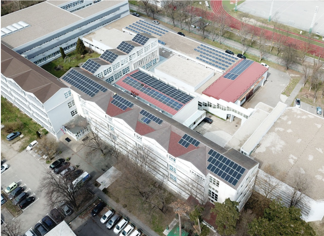
Figure 6.27 FERIT photovoltaic system modules on building roof in Trpimirova street
