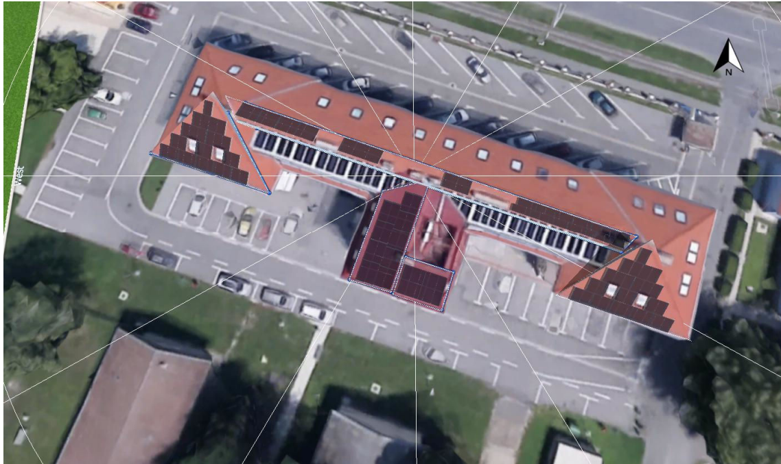
Figure 5.27 Preliminary 3D model of 35 kW PV system on building roof in Cara Hadrijana street
