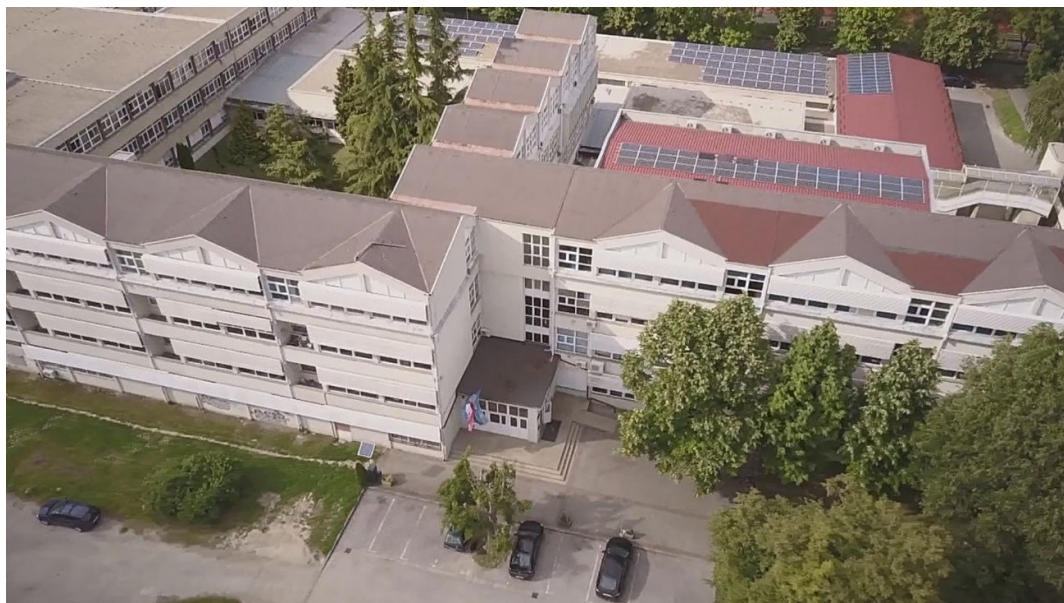
Figure 2.10 The main entrance to the building in Trpimirova street.
