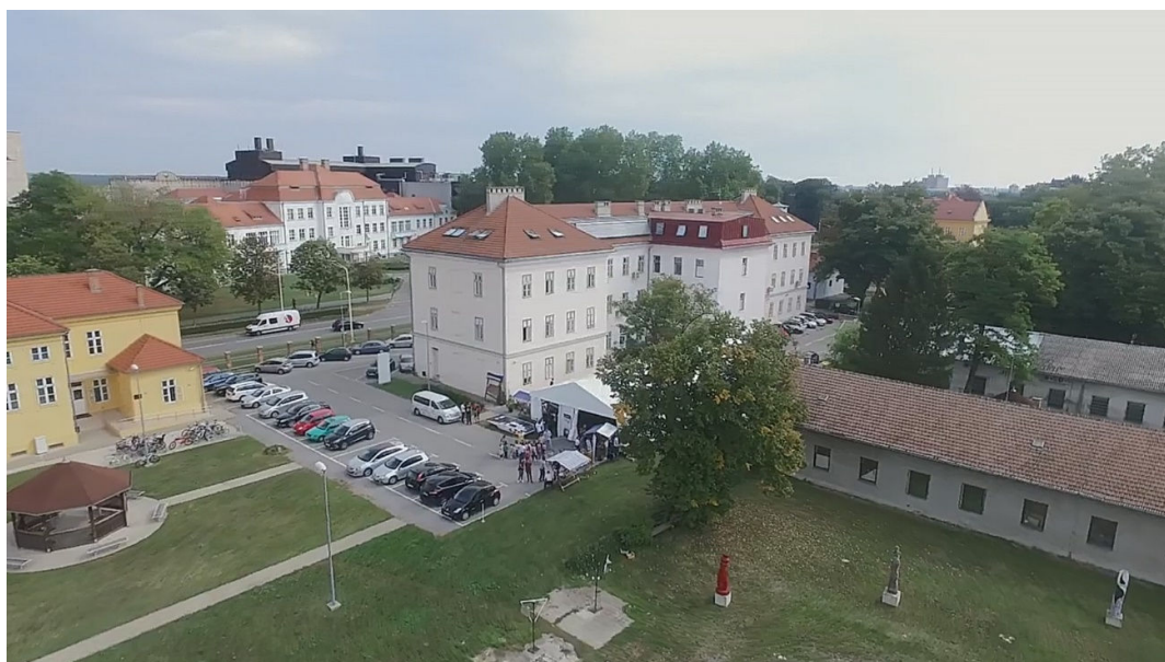
Figure 2.11 The main entrance to the building in Cara Hadrijana street.
