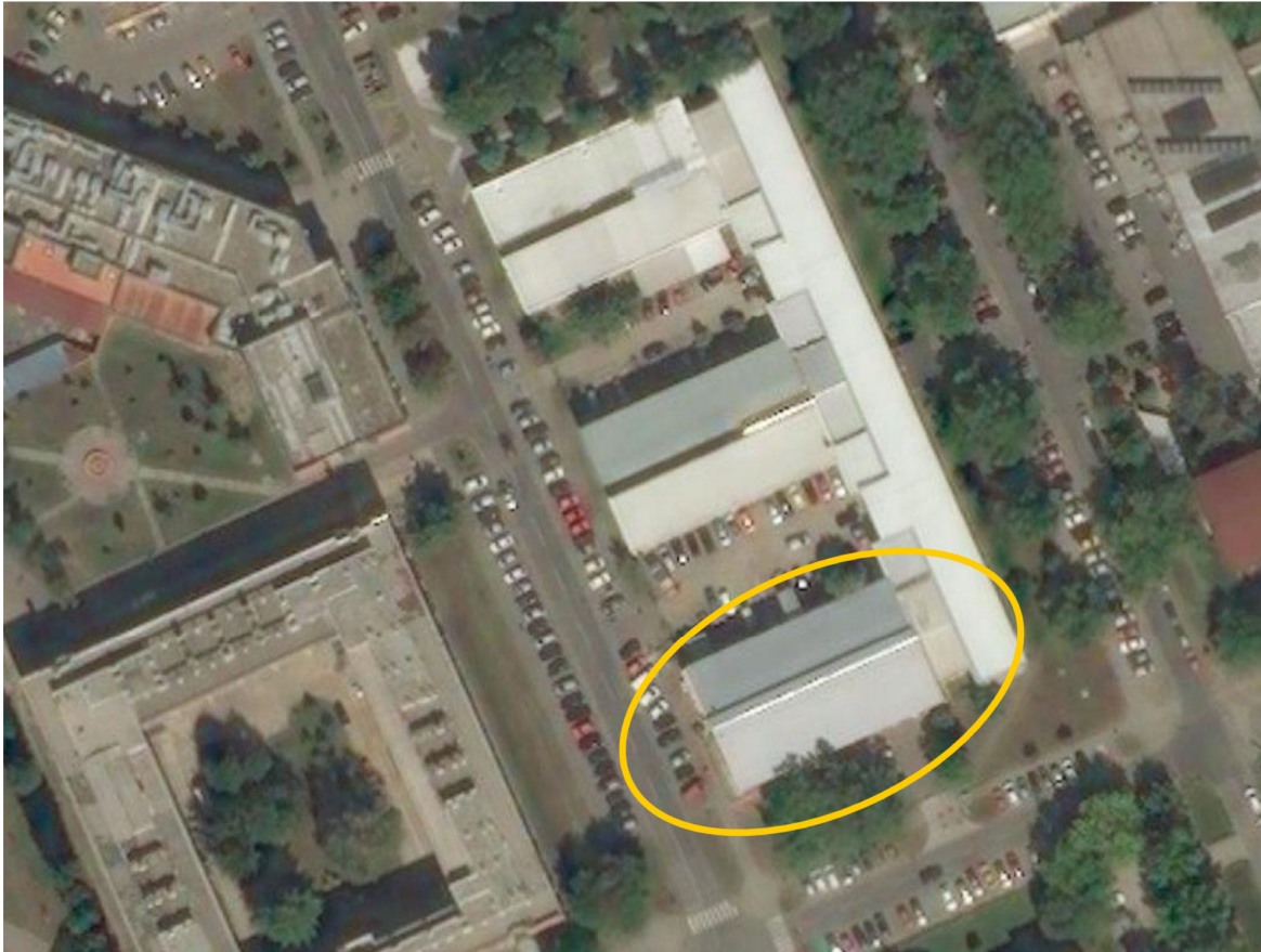
Figure 5.1 The location for the PV plant construction.
