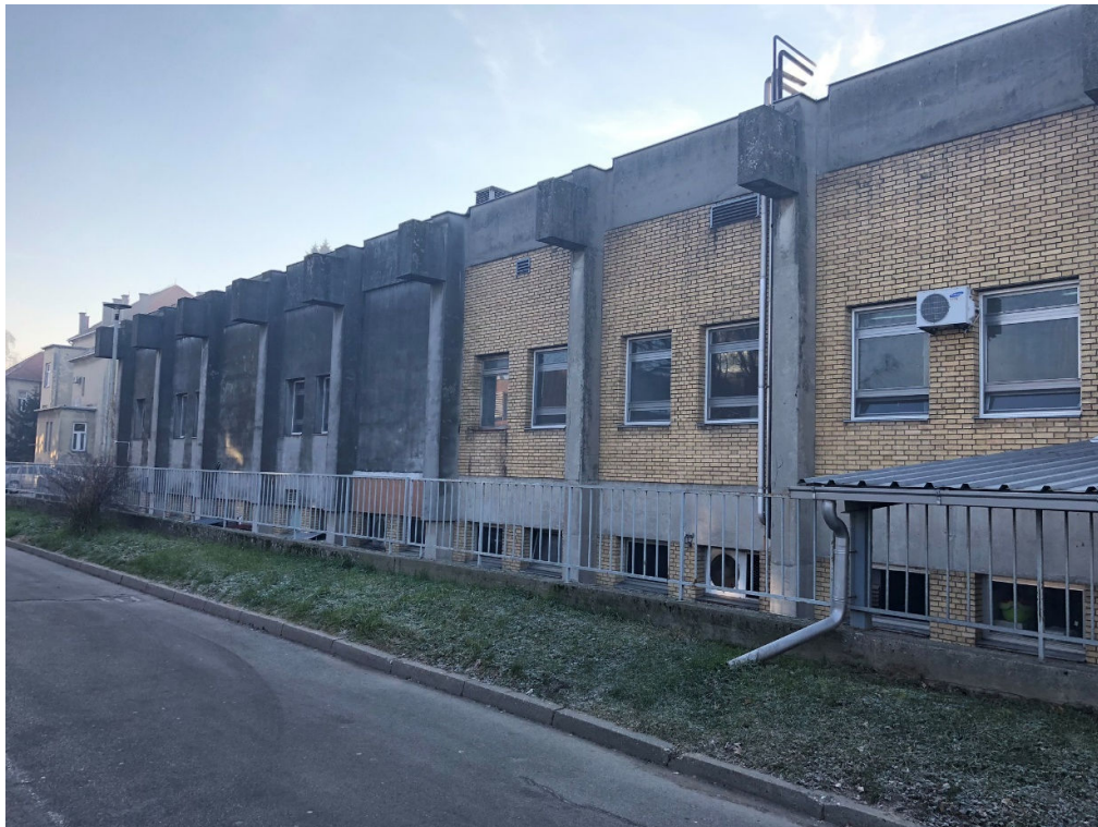
Figure 2.13 North side of the central kitchen building.
