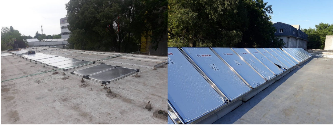
Figure 6.19 Solar-thermal system on the Medical Rehabilitation clinic roof
