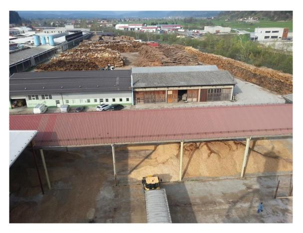
The main activity in the Biomass centre area of Nazarje is processing of wood for energy purposes. With powerful machines annually they produce approx. 170,000 loose m³ air-dried chips. With the completion of the investment, company provides an additional capacity of technically dried chips of 80,000 loose m³ per year and produced 3,000 tons of pellets. The processing of energy products is automated and operates 24 hours a day and employs 5 to 10 employees, depending on the season.
