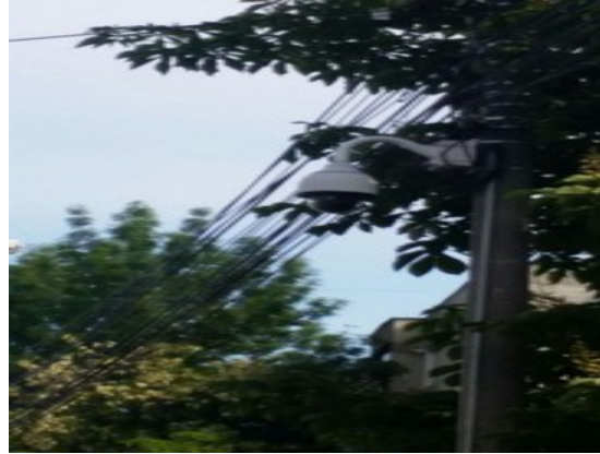
Figure 10 A surveillance camera for the traffic control system
