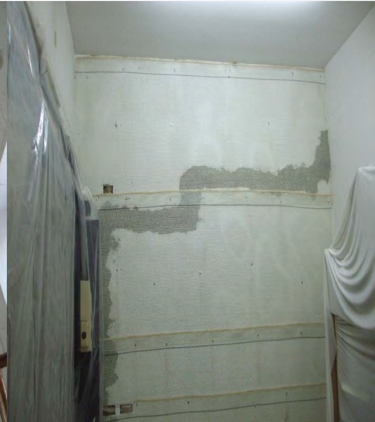
Repairing damaged house after earthquake
