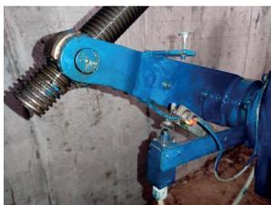
Limit switch on control arm of the turbine
