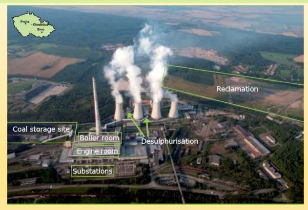
Installed power of 4x 205 MW and achievable power supply excessing 4 TWh per year
