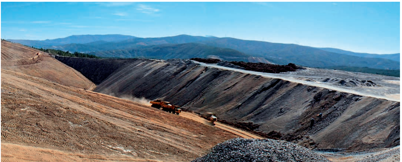
Ongoing construction of a new tailing disposal (October 2012)
