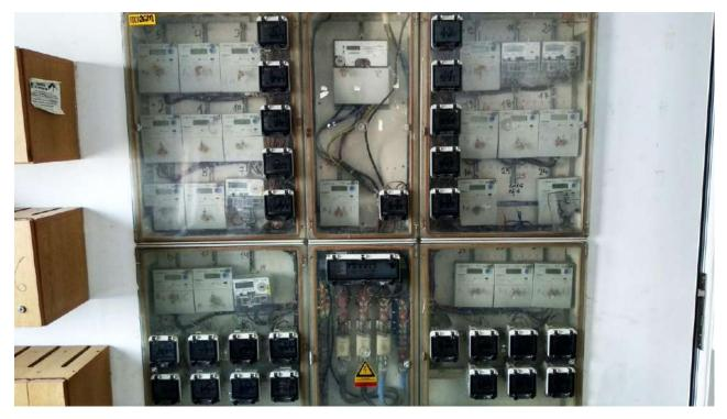
Fig. 8. General electric panel with fuses, protections, tri-phase general meter and individual meters (digital)
