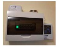
*Fig.* 5 – *Electricity fuse panel, Smart Electricity meter, climate unit and smoke detector*
