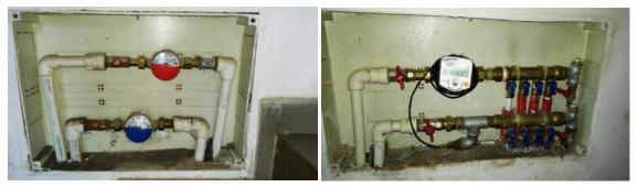
Fig.9. Cold and hot water meters
