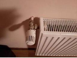
Fig.13. Radiator with mechanical thermostat
