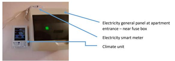
Fig. 3 – Electricity Smart Meter and Climate (Temp, Humidity, CO2) unit with display
