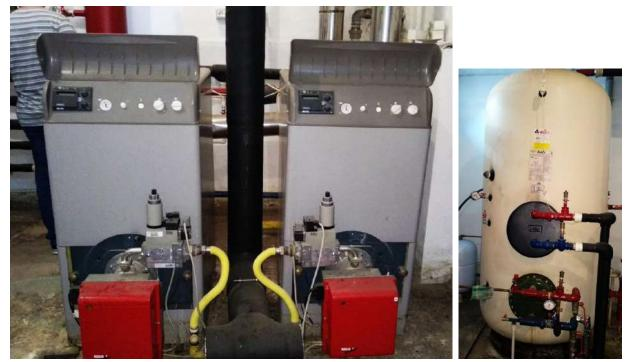
Fig. 6. Heating/ boiler systems for heating and hot water;
