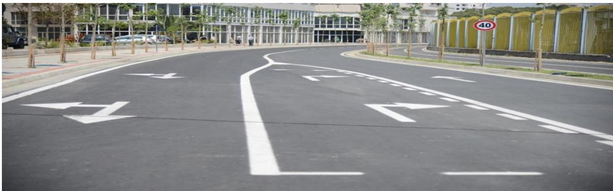
The first part of the road from "DAJLAN BRIDGE" to the ferry shore is designed as a 2-lane road, 1 bicycle lanes with a total width of 10.5m, with the passing width of  $B = 7\text{m}$ .
