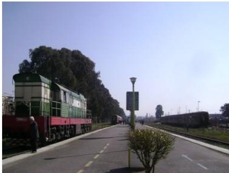
Figure 6 - Durrës railway Station
