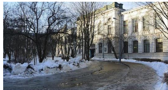
Figure 5. SPbPU Chemical Building at present time
