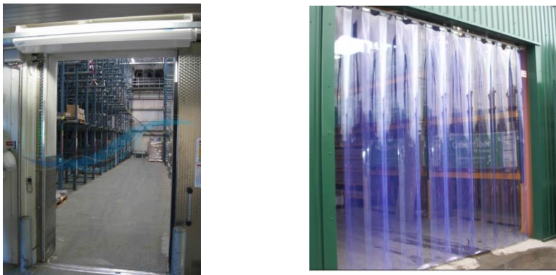
Figure 38: Air curtain and plastic slat curtain used in cold storages
