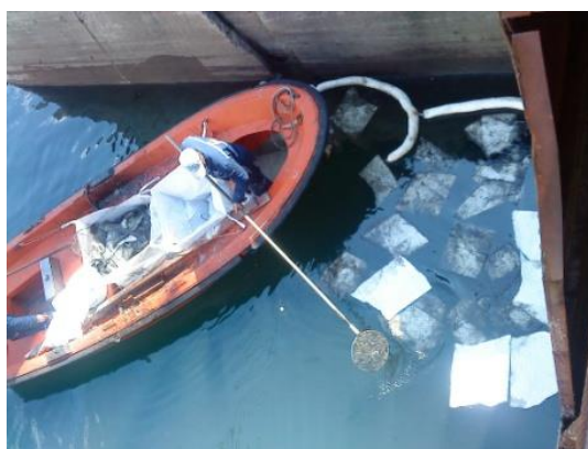
Picture 2.12: Response to an oil pollution incident by using absorbents and floating barriers within the PPA SA port area
