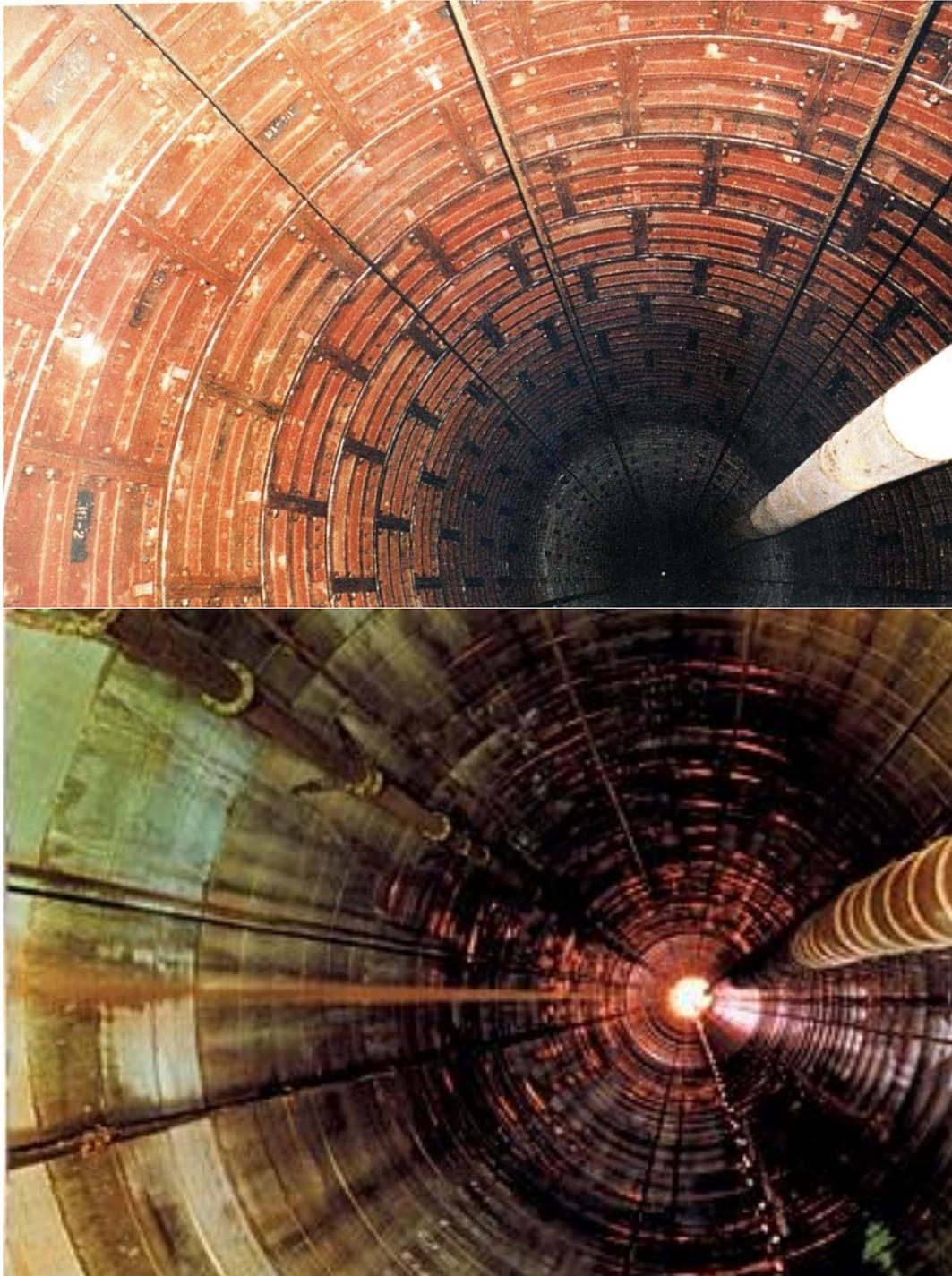
Figure 3.11. An example of the shaft with the iron cast (above) and concrete lining (down)
