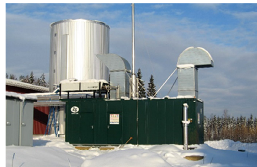
Photo 1, 2. Juvan Bioson OY Production Buildings. Photo: Hanne Soininen
