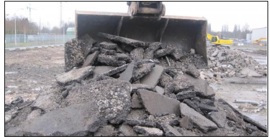
Asphalt with high % recycled materials
