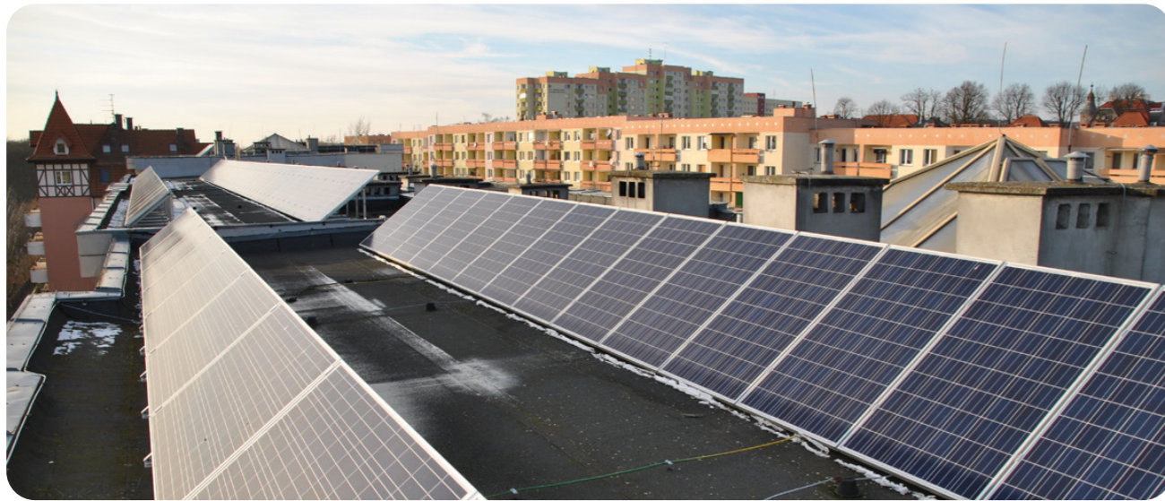
Pszczelna Solar Housing. Photo: Krzysztof Stasiewicz
