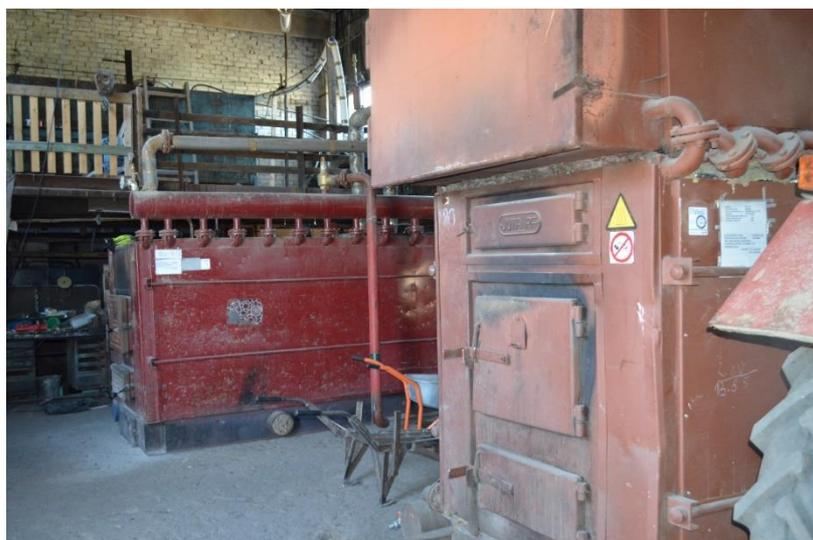
Fig. 3.4.1 Wood boilers with capacity of 1 and 1.5 MW installed in Lejasciems boiler house
