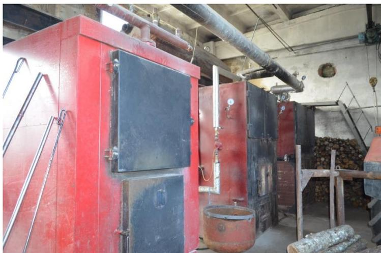
Fig. 3.2.1 Wood boilers installed in the boiler house
