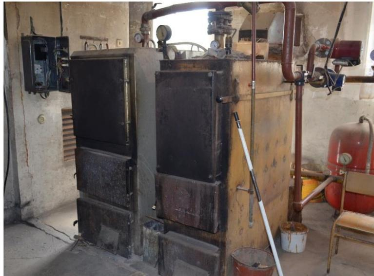
Figure 3.6.2. Boilers installed in the parish administration building
