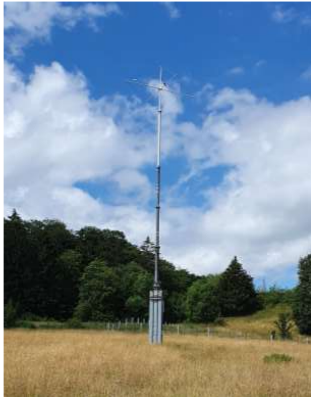
Figure 11 Typical MF antenna used on German R-Mode/DGNSS sites (Typ NTA, Koblenz DGNSS)
