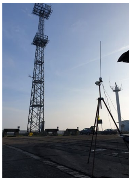
Figure 6-13: Photo from measurements d)
